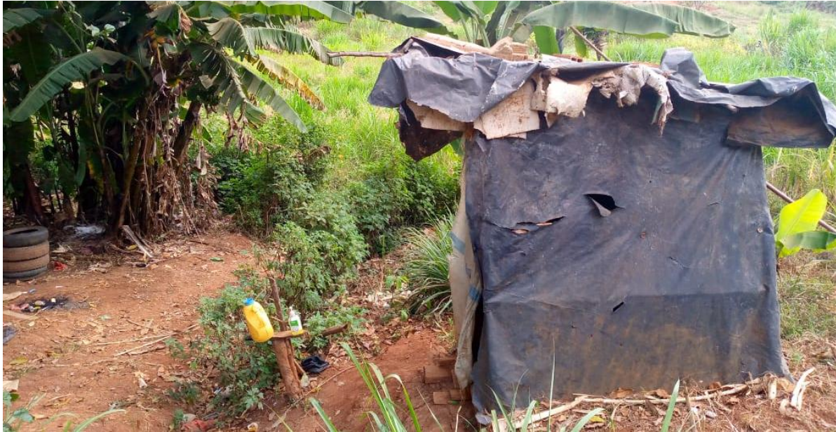
Figure 10 Temporary Pit Latrine Located 5 Metres from River
