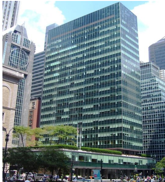
Fig 4: Lever House, New York (G Bunshaft & N. de Blois, 1952)
