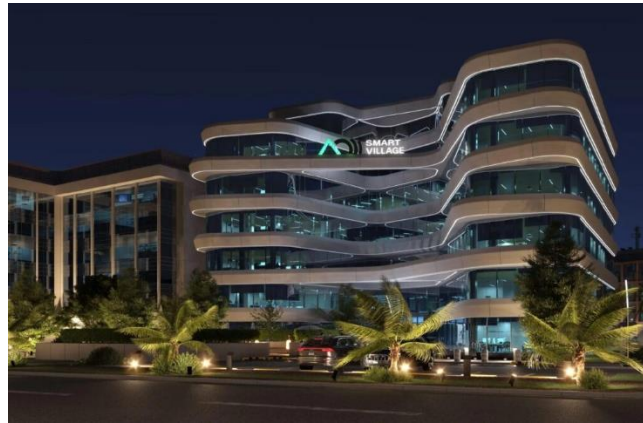
Fig 14: Smart Village Office Buildings, Cairo, Egypt - showing recessed facades and shading screens that are employed to minimize the amount of sunlight exposure.
