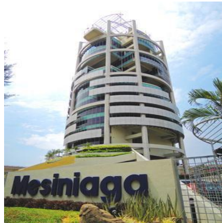
Fig11: Ken Yeang. (1992). Menara Mesiniaga, Subang Jaya, Malaysia - with external shading fins and sky garden terraces incorporated in the building envelope. Retrieved from CTBUH / architectural archives.
