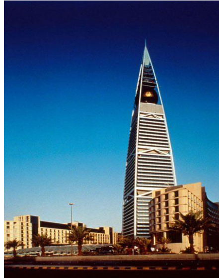
Fig 12: Foster + Partners. (2000).: Al Faisaliah tower, Riyadh, Saudi Arabia - shows how the reflective curtain wall facade is used to reduce solar heat gain. Retrieved from architectural archives / CTBUH.
