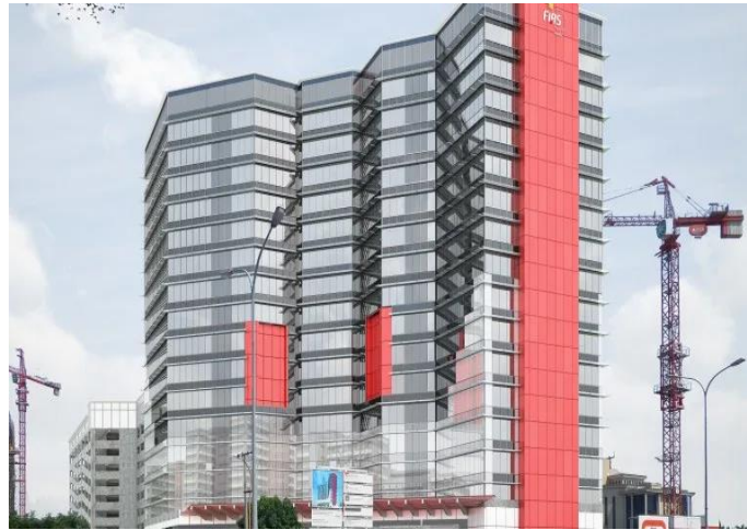
Fig 8: Federal Inland Revenue Service Headquarters curtain-wall façade and multi-tower configuration.
