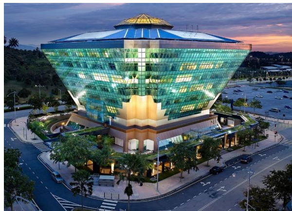
Fig 10: Diamond Building (Energy Commission Headquarters), Putrajaya, Malaysia - the depiction of the self-shading building geometry and facade shading designs. source: (NR Architect, 2010)
