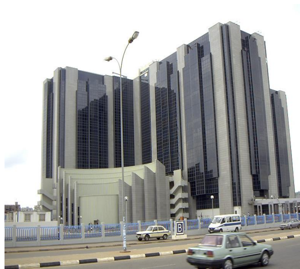
Fig. 7: Central Bank of Nigeria Headquarters, Abuja, showing the deep-set punched-window façade system.
