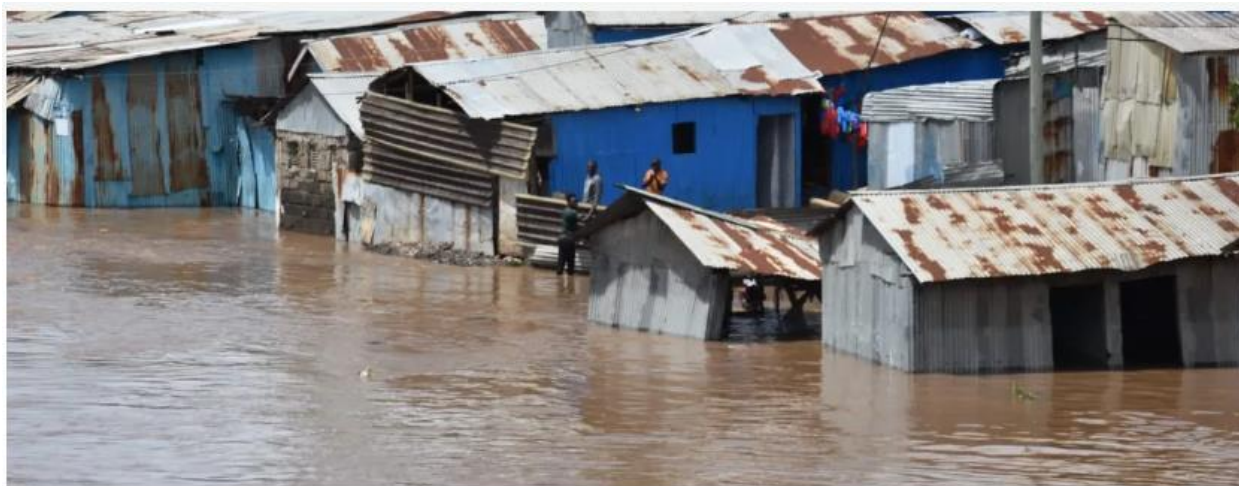
Figure 25 Flooding incidence in Mukuru Viwandani Source: ©Shakur Njeru, Viwandani Comprehensive Community Organization (VICCO), 2024
