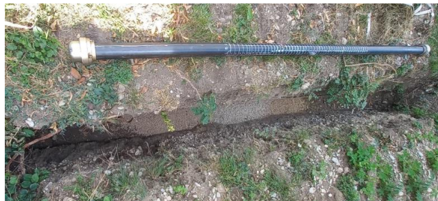
Figure 11. Pipe in the preliminary stage of installation in the trench
