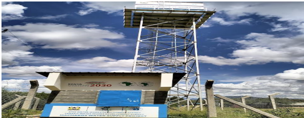
Figure 10: Borehole by Athi Waterworks Development Agency at Makyau. Source: Author 1 2024.
